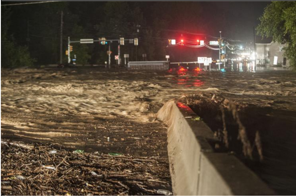
Figure 4.3.3-4 Flood waters rushing across Rt. 119 in Connellsville City, Fayette County 2016 ( heraldstandard.com , 2016)
